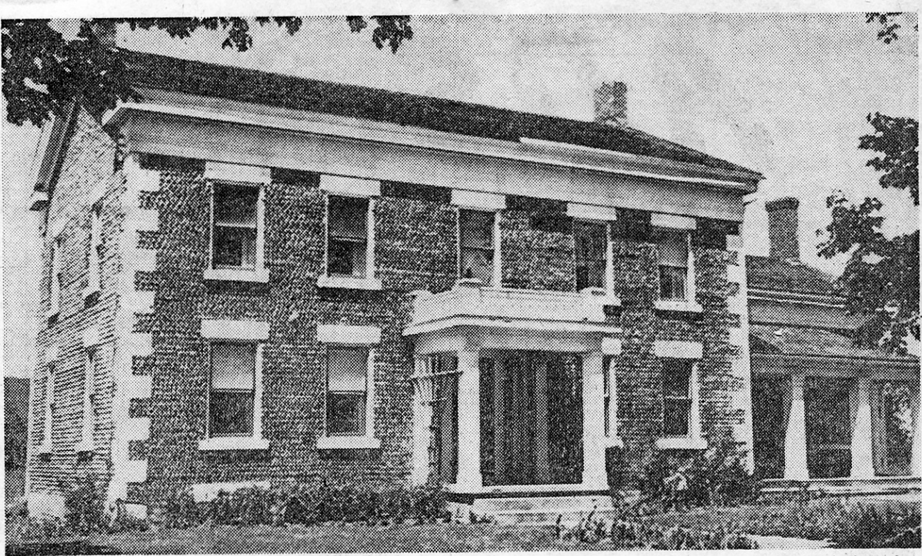
ON FAMOUS SITE —This cobblestone house on hill in Maple Road, short distance north of Palmyra, was built in 1849 after original Martin Harris house burned.
